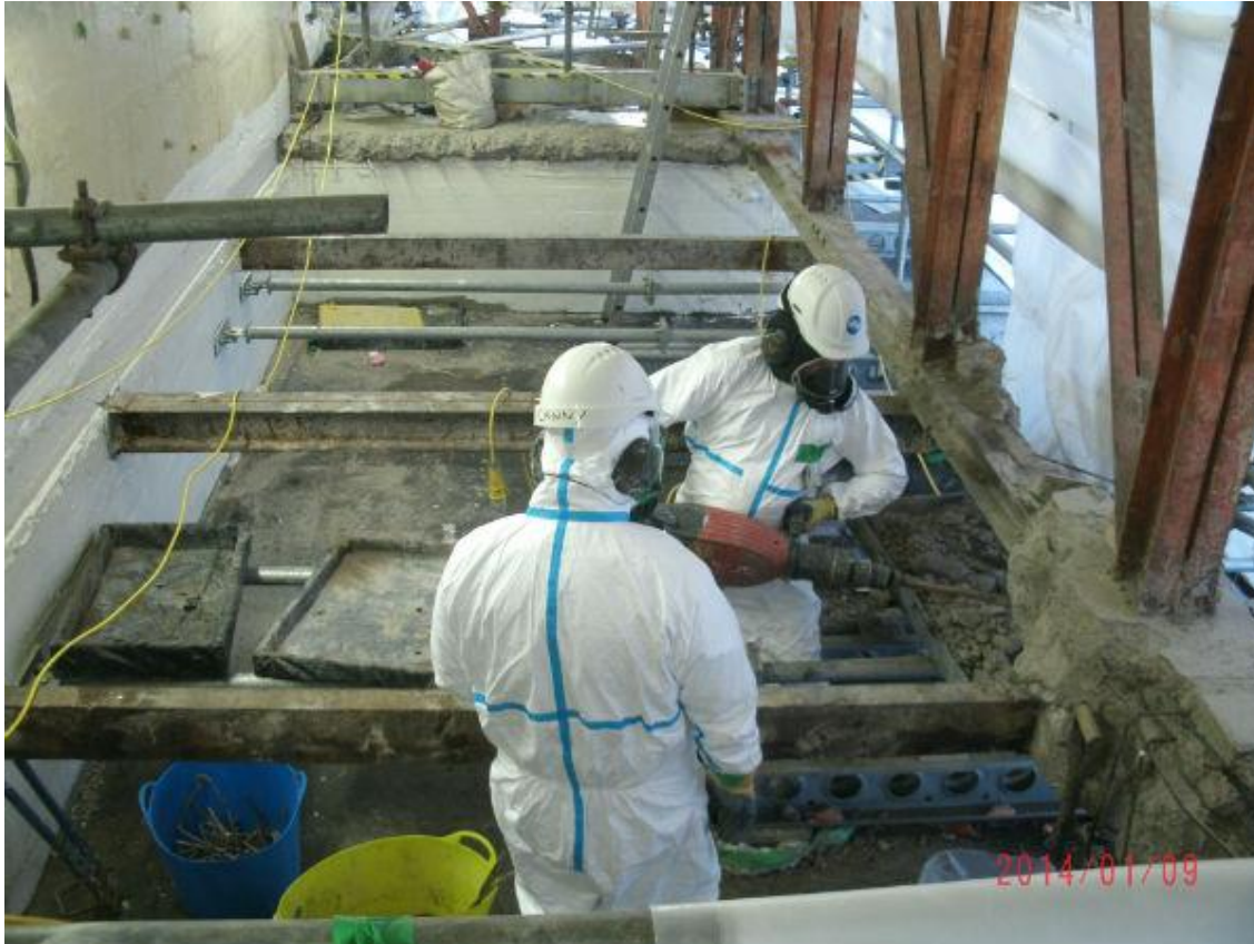
Windscale pile filter decommissioning, Nuclear Engineering International
